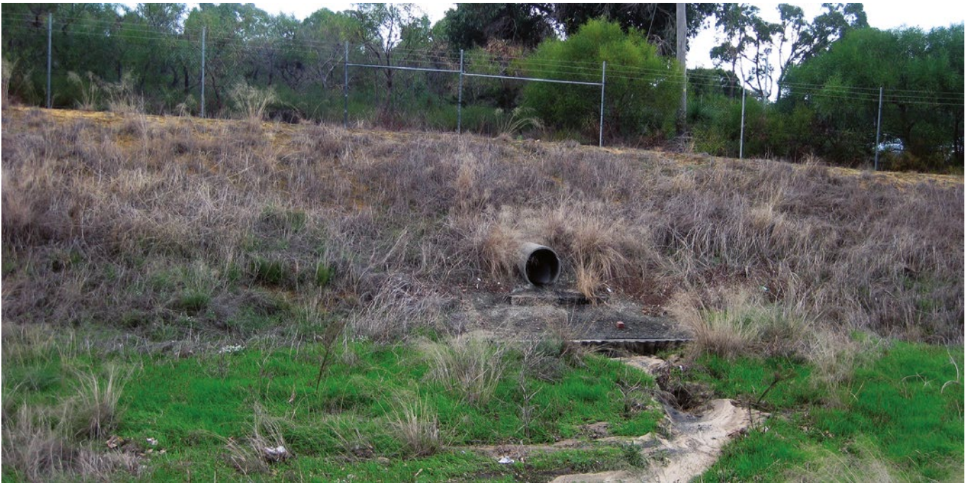
Figure 22: Fenced Off Sump at Lilburne Park
