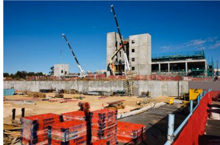
Photo: Construction site in Joondalup
