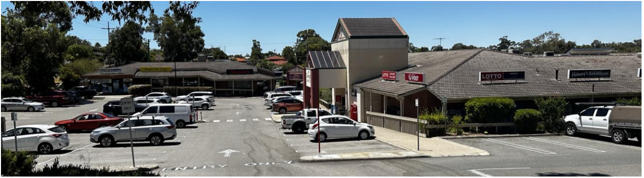
FIGURE 1.1. GLENGARRY SHOPPING CENTRE (JANUARY 2024)
