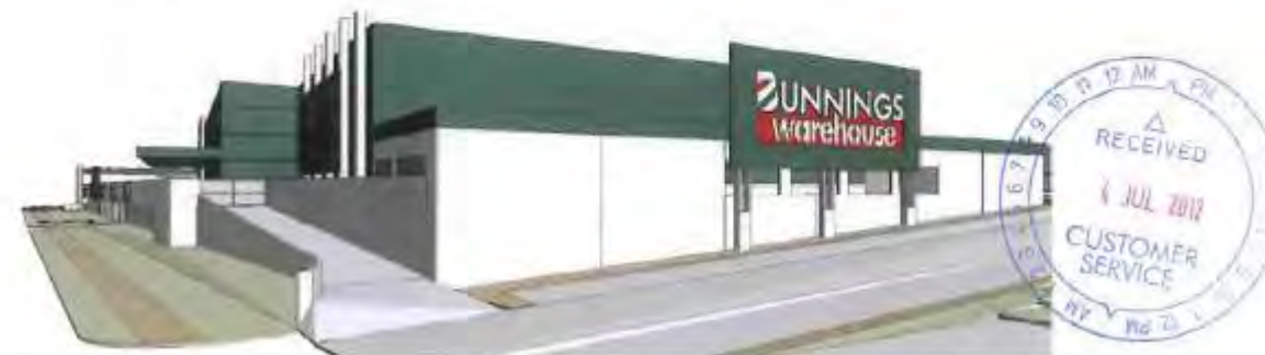
South East Ramp Off Honeybush Drive
