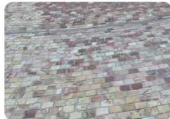
INTIMATE PAVED DETAIL AREAS
