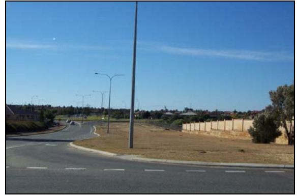
Photo 2: Boundary of Lot 9019 looking north along Connolly Drive.
