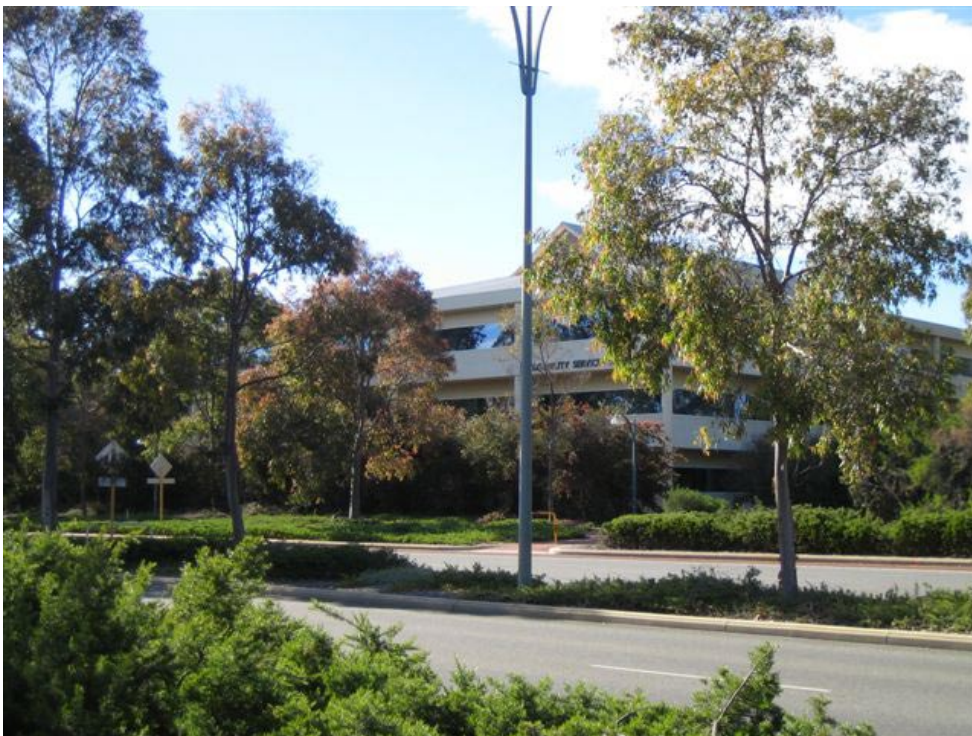
Photo 4 - Existing office building viewed from Shenton Avenue (Note: Width of carriageways.)
