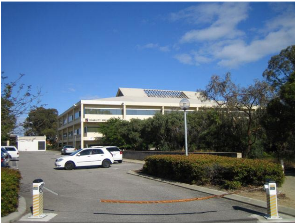
Photo 2 - Existing office building and car park
