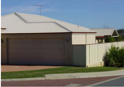
Photo 1: Unacceptable corner treatment
