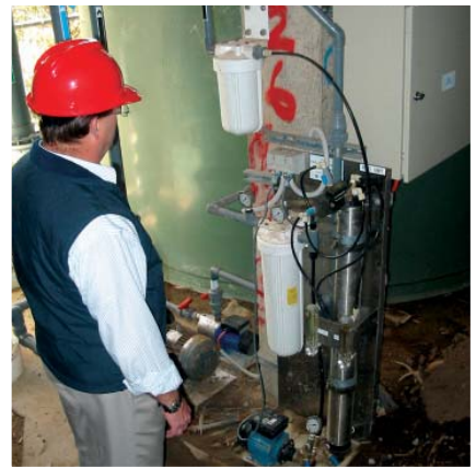
Ross McPherson, Manager-Water Catchments, Hornsby Shire Council, New South Wales, Reverse Osmosis Filtration Unit at Hornsby Aquatic Centre. This initiative is included in Hornsby Shire Council's Milestone 3 Local Action Plan.
