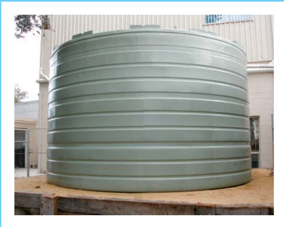
Collected rainwater is used for plant irrigation and is estimated to reduce consumption by 350–400 KLs per annum. Irrigating open space was identified as a major water using activity by Frankston City in Milestone 1. The above photo of a 45KL holding tank was provided by Frankston City, Victoria.
