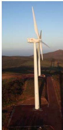
Wind turbines in the Galapagos
