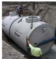
Rain vault installation
