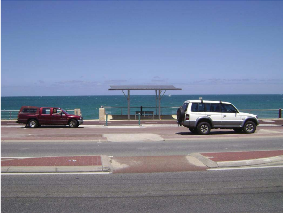
Shade structure opposite Ross Avenue, Sorrento.
