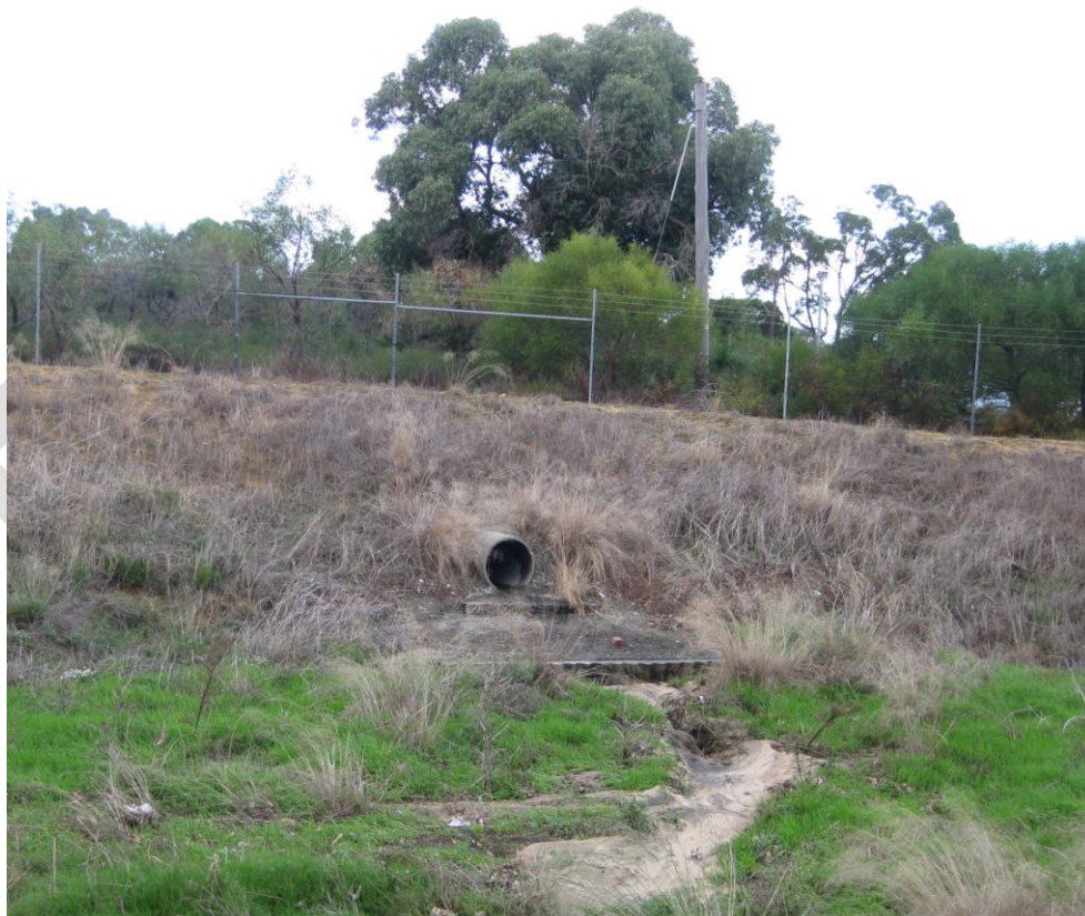
Figure 22: Fenced Off Sump at Lilburne Park
