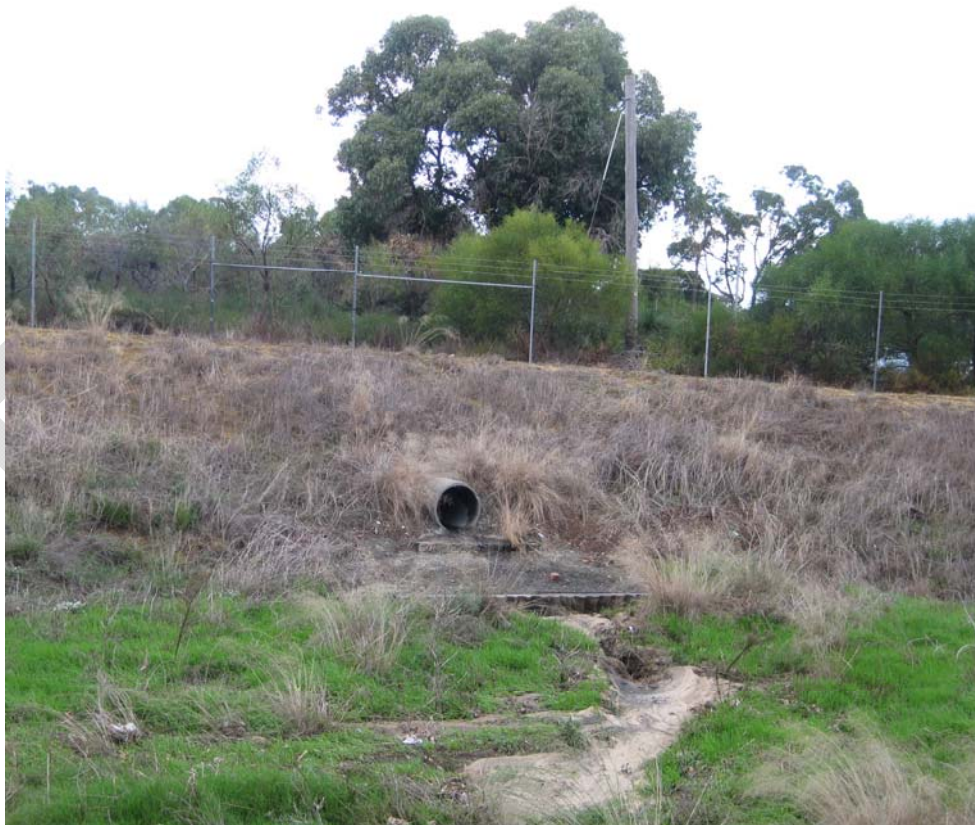
Figure 22: Fenced Off Sump at Lilburne Park
