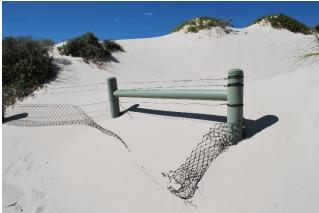
Figure 6: Erosion along the foredunes and beach affecting stability of fencing
