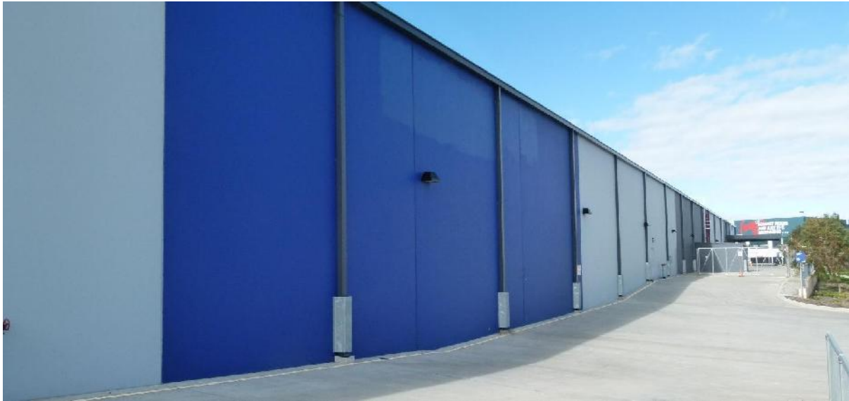
Photograph 4: View of rear of subject site looking east.
