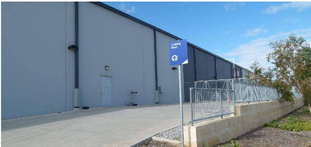
Photograph 5: View of rear loading dock, looking east.
