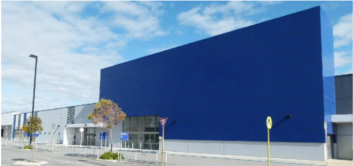
Photograph 1: Former Masters building façade and car parking area.
