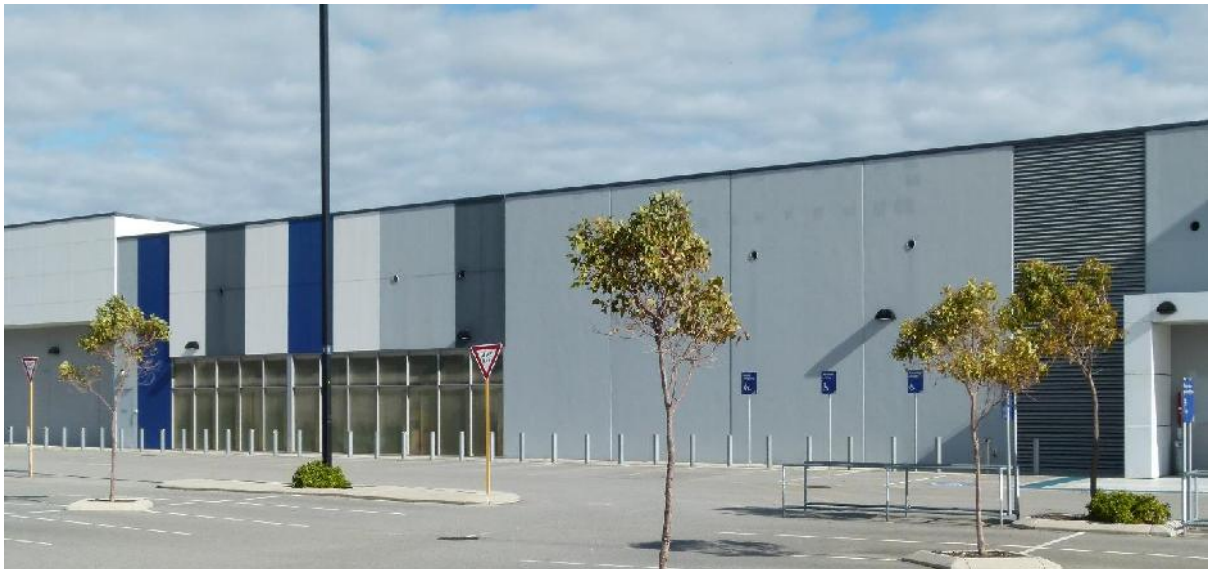
Photograph 2: Former Masters building façade and car parking area.
