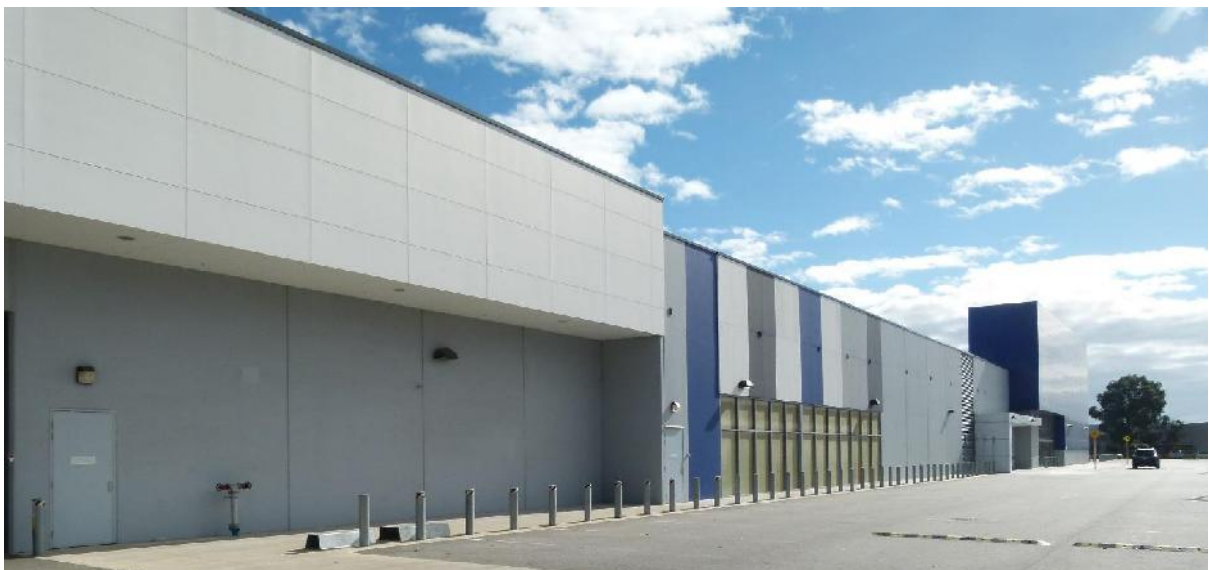
Photograph 3: Former Masters building façade and car parking area.
