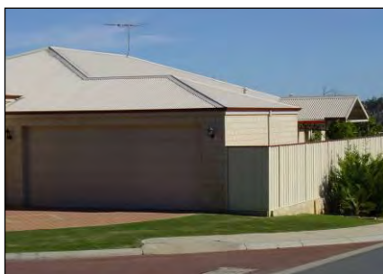
Photo 1: Unacceptable corner treatment
