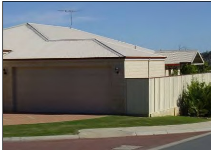
Photo 1: Unacceptable corner treatment
