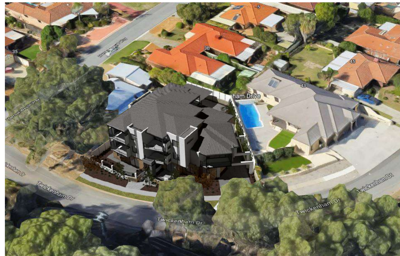
ILLUSTRATION - OVERVIEW FROM WEST NORTH-WEST
