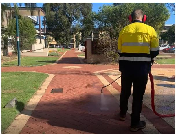
Figure 15: Photograph of the City's chemical-free weed control in July 2022
