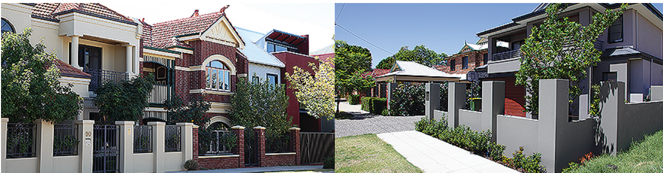
Figure 38 High street walls should be limited to the minimum necessary and be visually permeable
