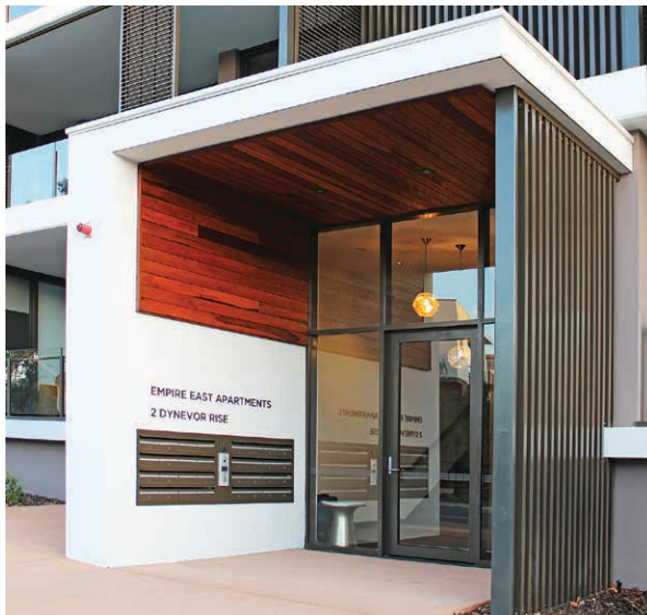
Photo G2.7a This development, designed for adaptability and universal access, has a considered entry sequence with a wide, obstacle free path to the entry
