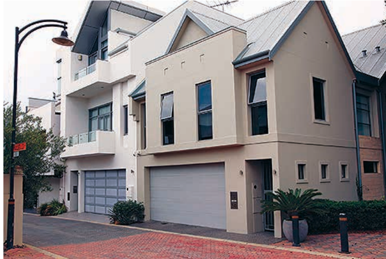
Figure 42 Garage doors, particularly on narrow lots, can be an imposing element in the streetscape
