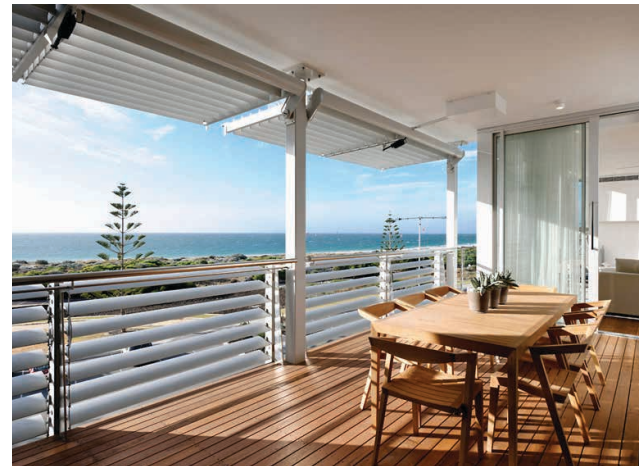
Photo G2.2a Adjustable louvres are an effective way to control sun, glare, privacy and ventilation through the day and year (PC)
