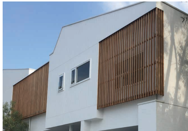
Photo G3.10b The privacy screening on this development has been effectively integrated into the building design
