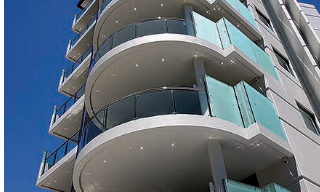
Screening devices used to provide for increased visual privacy between developments.
