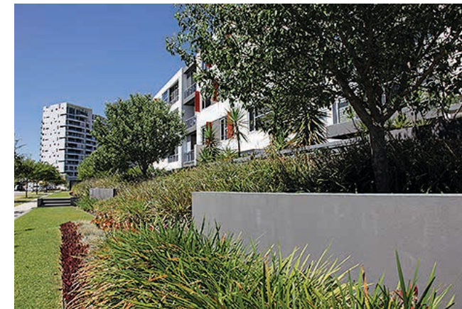
Landscaping enhances outlook from apartments as well as facilitating stormwater infiltration.
