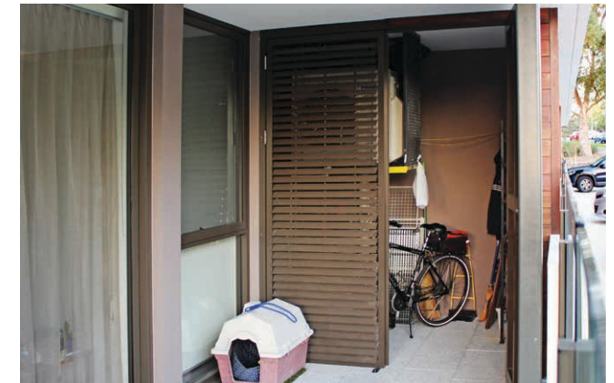
Photo G2.1b and c This storage area has been neatly integrated into the design of the balcony, is conveniently located, is of useful size and proportions, weatherproof, and screened from view.
