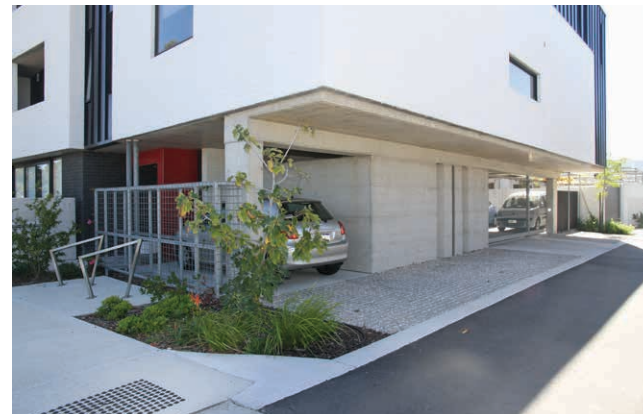
Photo G2.3a Undercroft parking reduces the visual impact of parking on the street and provides an opportunity for flexible use of the space when not required for car parking
