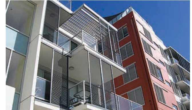
Screening devices used to limit views between internal spaces of one dwelling and the balcony of the adjoining building.
