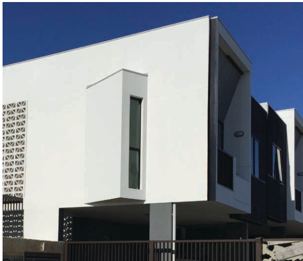
Photo G3.10a The upper level windows on this apartment have been oriented toward the communal space to help address visual privacy
