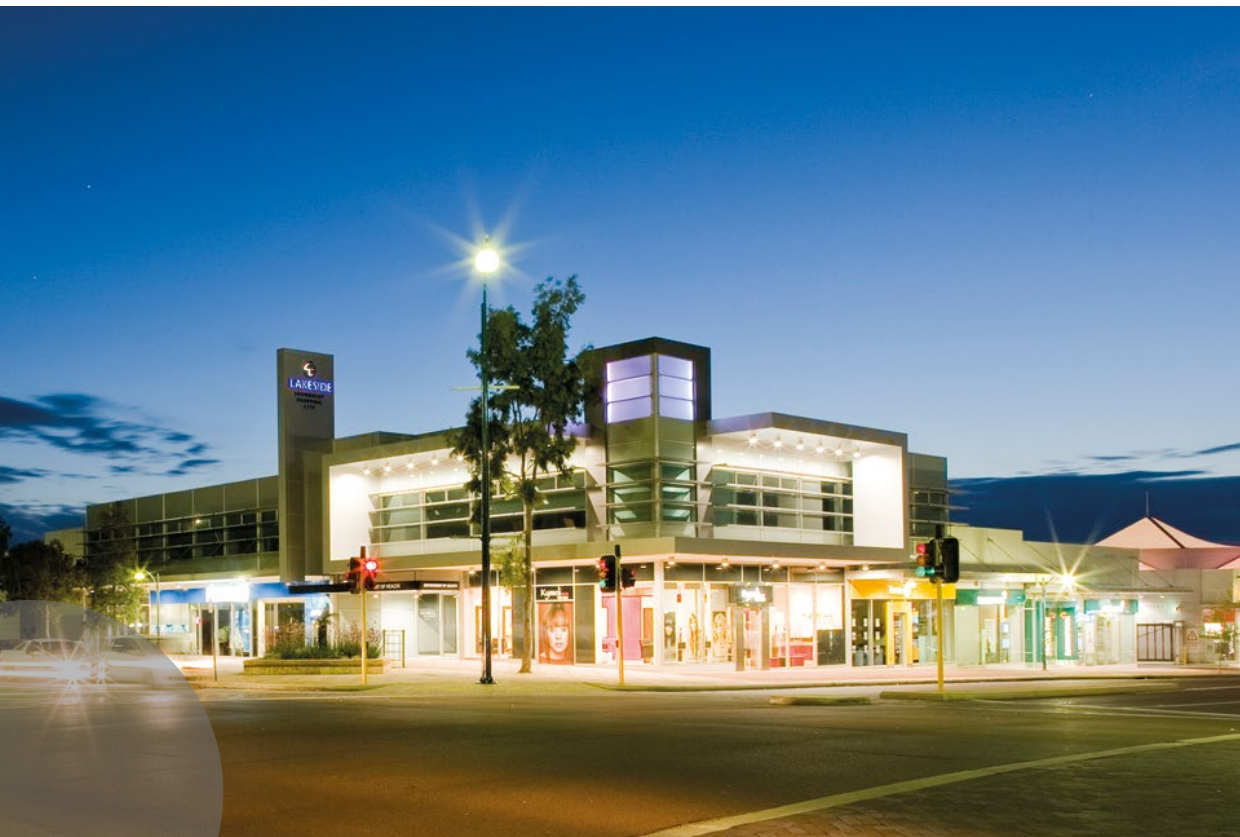
Lakeside Joondalup Shopping Centre – image courtesy of Greg Hocking
