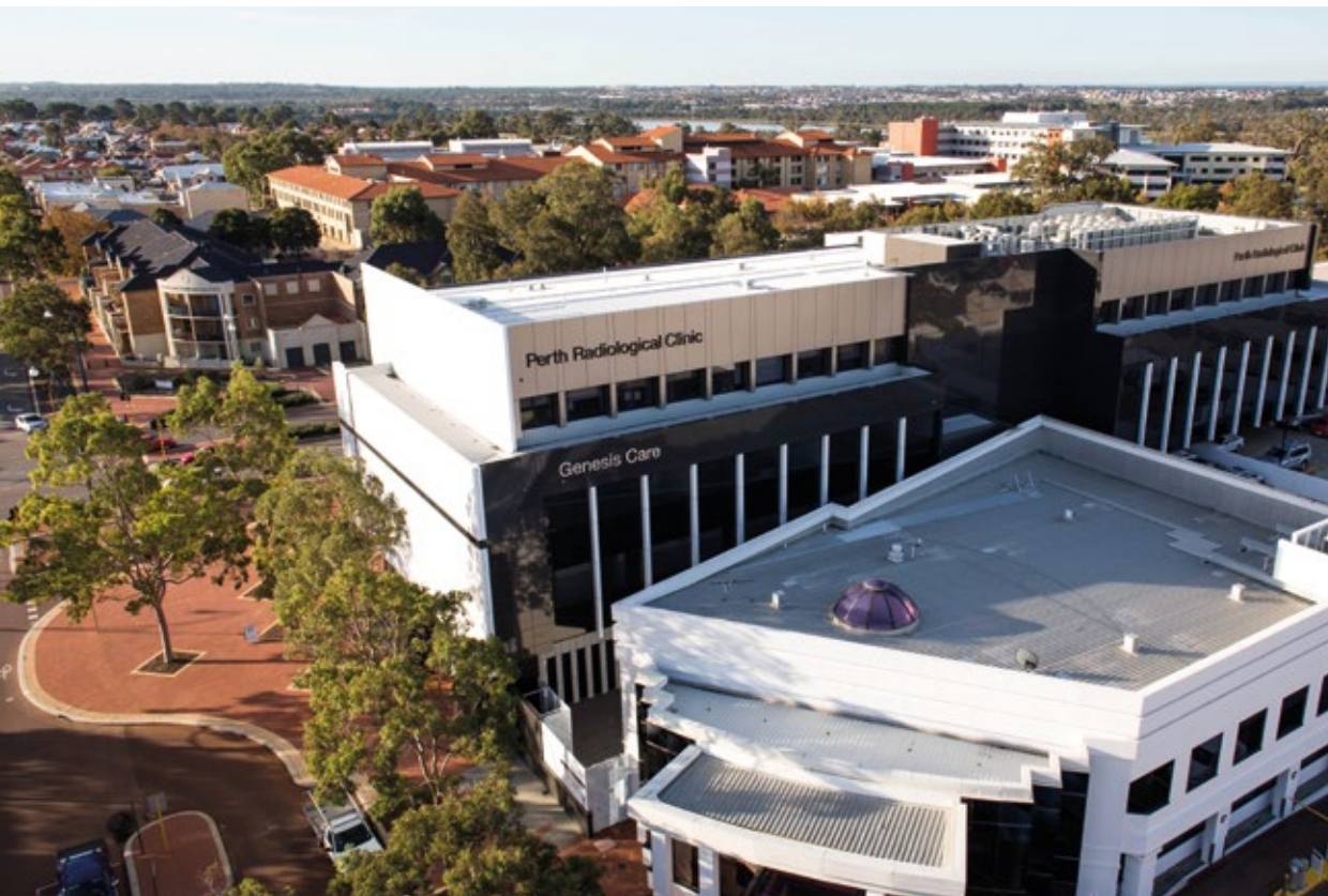
Shenton House and Joondalup Health Campus
