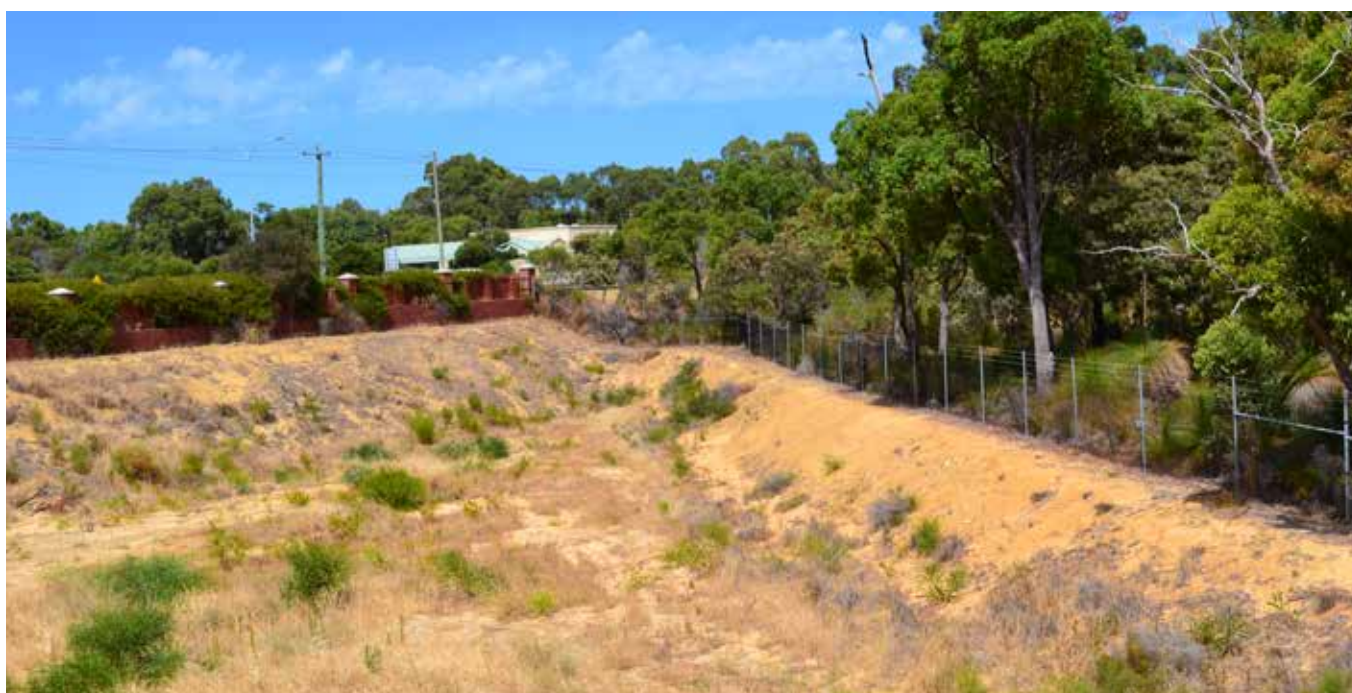
Figure 30: Fenced off Sump at Hepburn Heights
