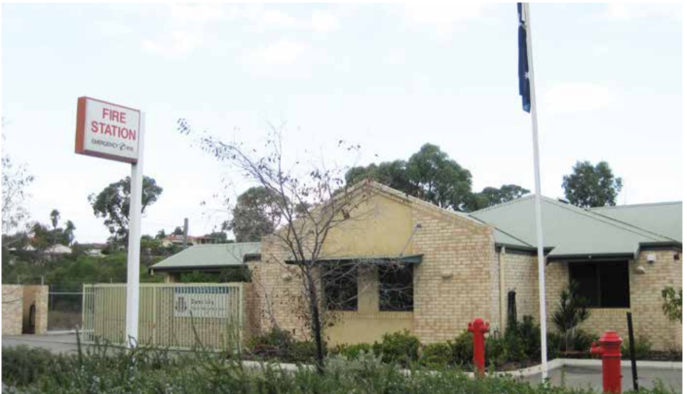
Figure 33: Duncraig Fire Station
