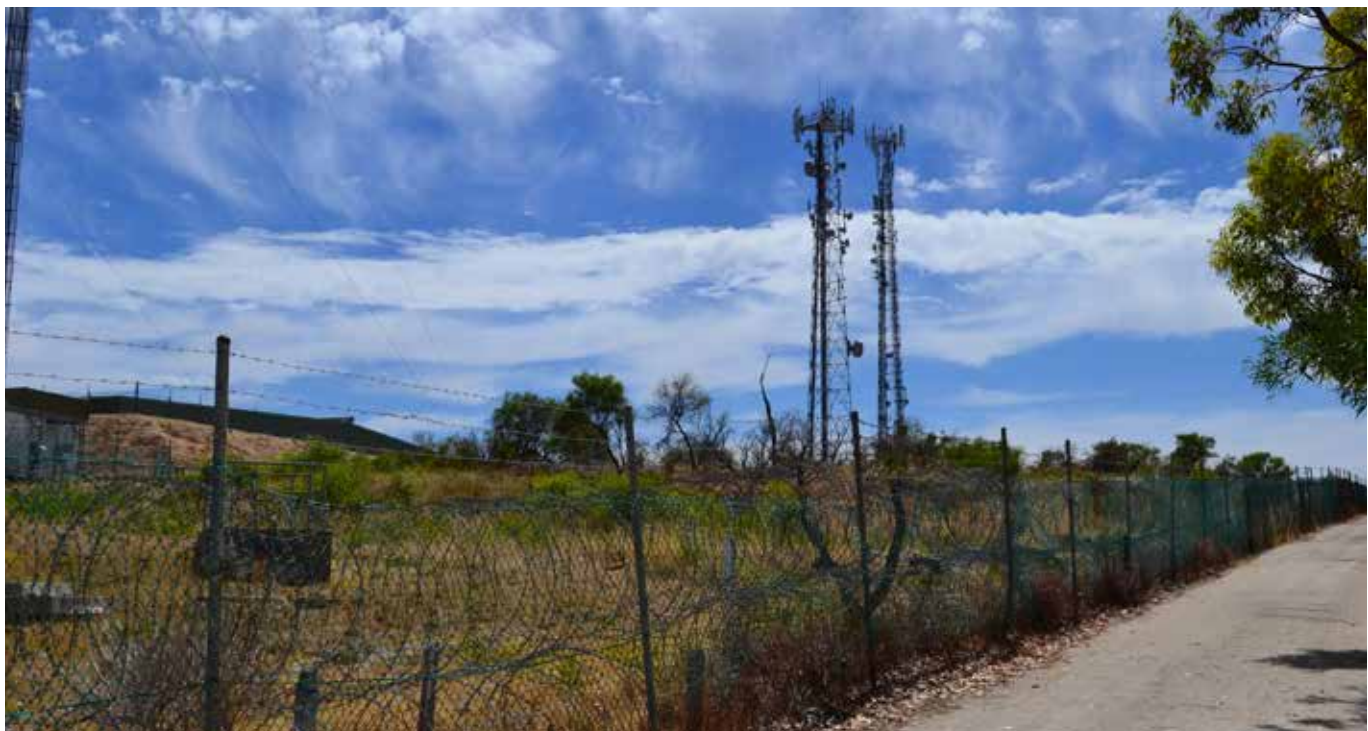
Figure 32: Water Supply and Telecommunications Facility
