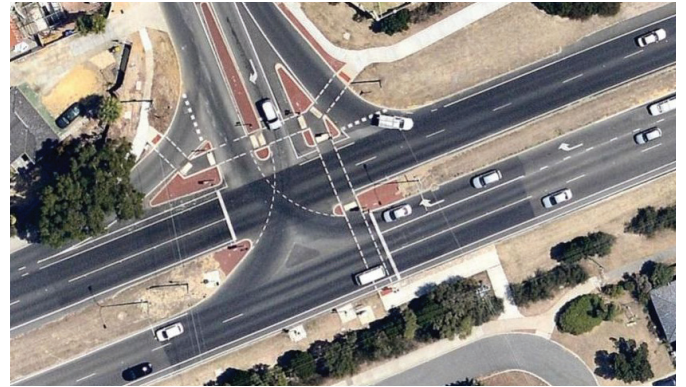
Image: Whitfords Avenue and Eddystone Avenue intersection post construction.
