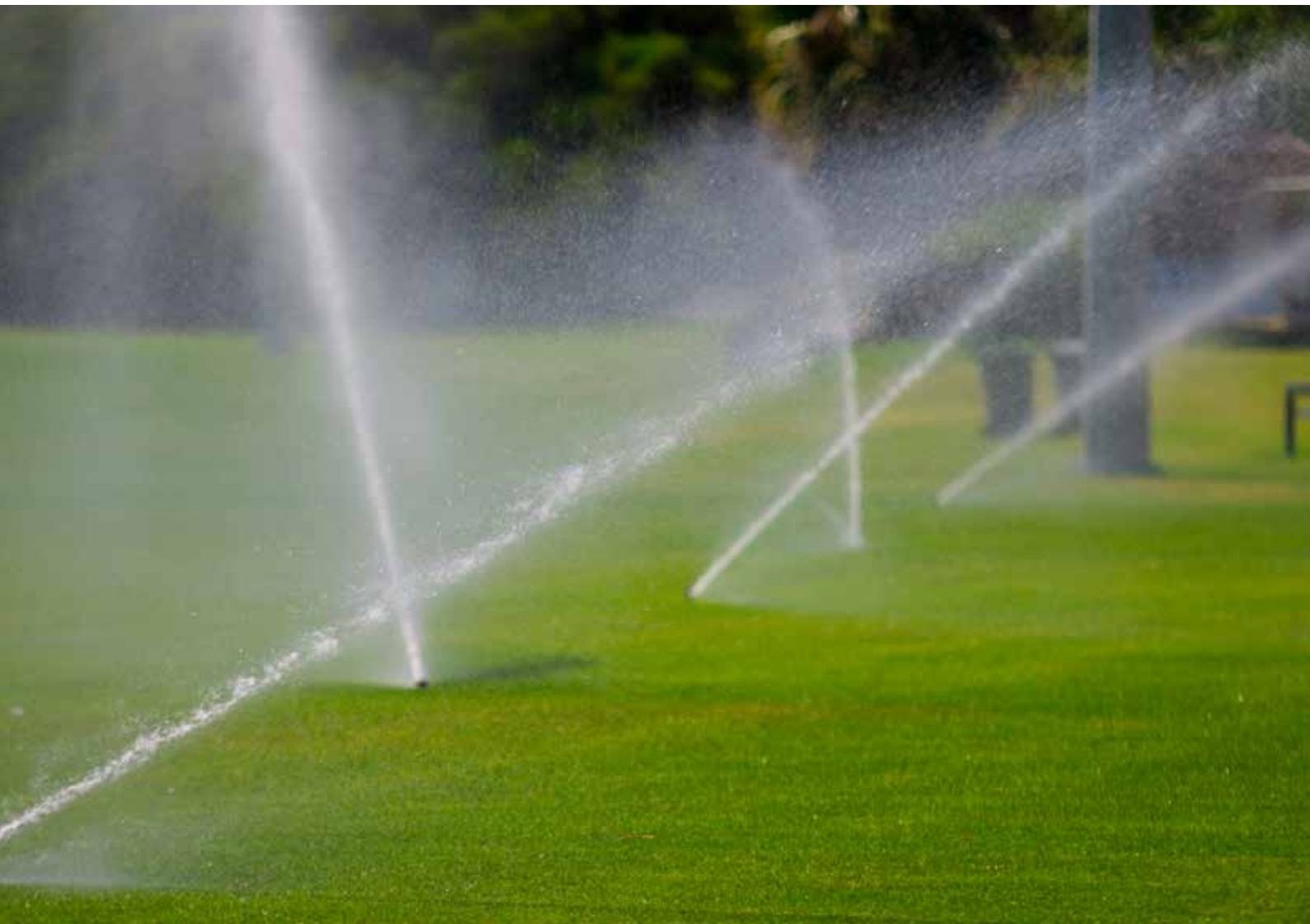
Irrigation testing at Iluka District Open Space (Currambine)
