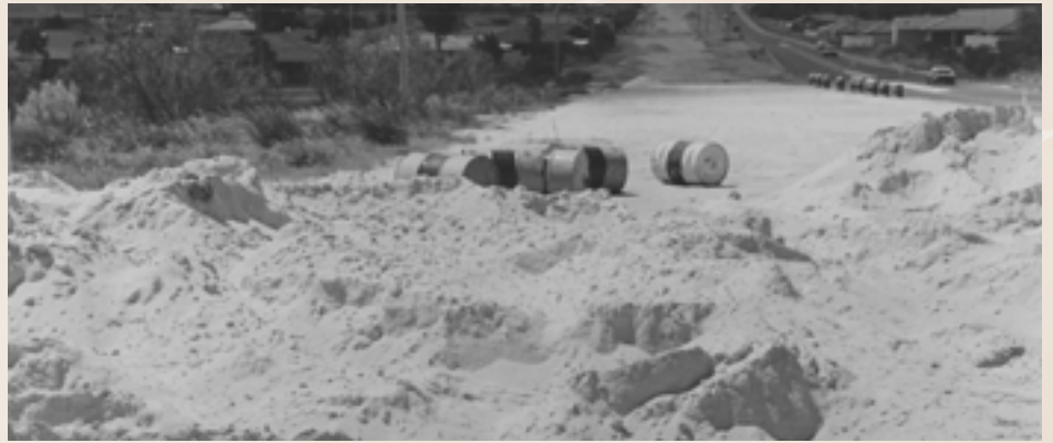
Digging Ocean Reef Road, Heathridge ca.1987.
