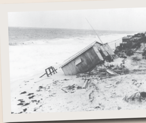
Whitford shack after storm damage ca. 1964.
