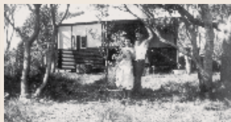
George and Joyce Sears pictured in front of their newly built house, ca. 1935.
