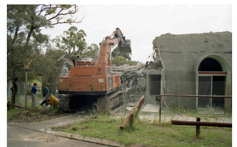
Demolition of the Greenwood Binishell 3 October 1989.
