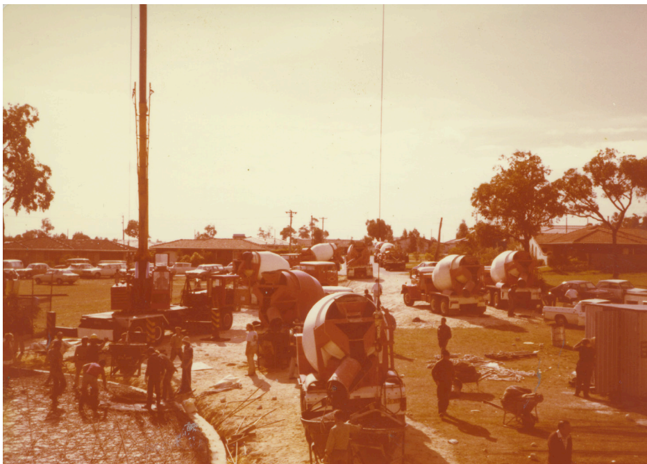
Construction of the Greenwood Binishell, Penistone Reserve Greenwood, 1977.
