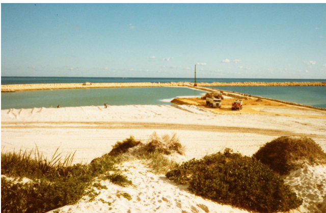
Hillarys Boat Harbour under construction (1986)
