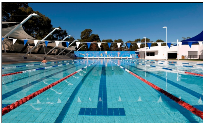
Outdoor 50 metre swimming pool at Craigie Leisure Centre which utilises geothermal heating (May 2011)
