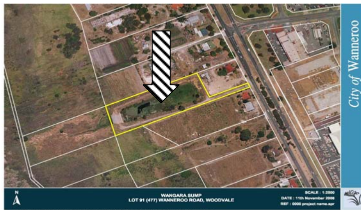
Figure 12. Aerial photo of the Wangara sump, which receives untreated stormwater from the Wangara industrial area.
