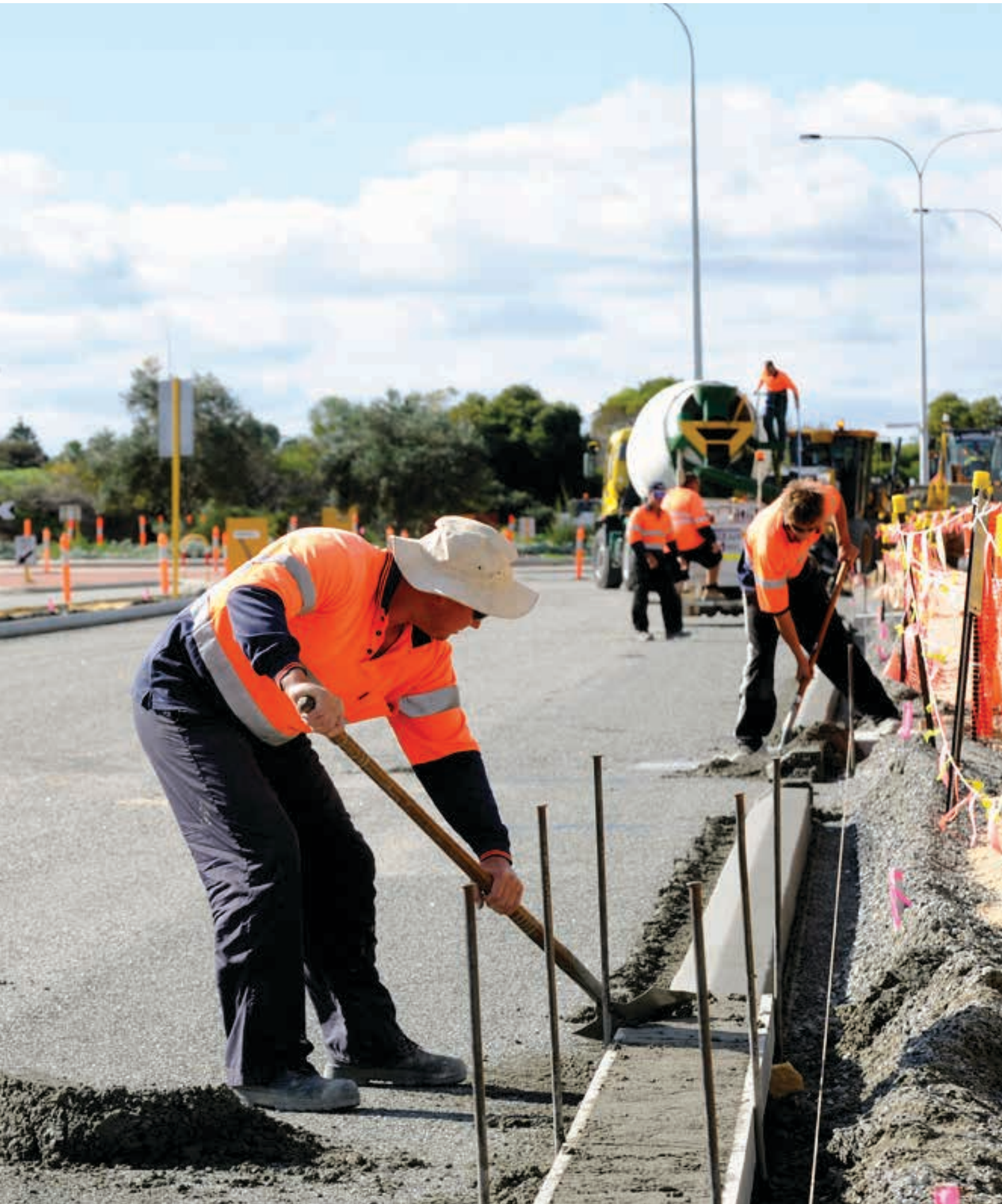
Shenton Avenue/Moore Drive upgrade
