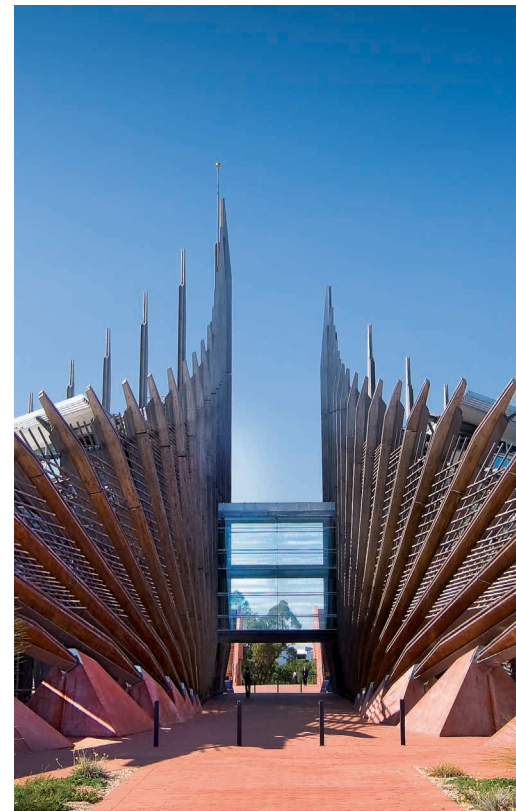
ECU's iconic Chancellery Building
