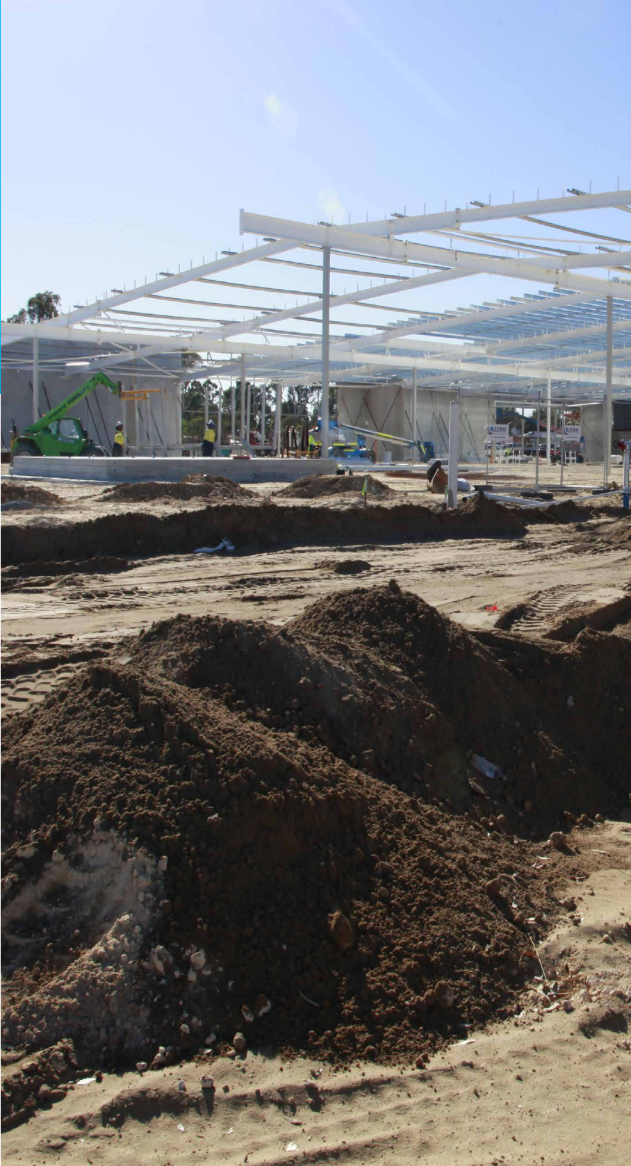
Joondalup Quadrangle construction
