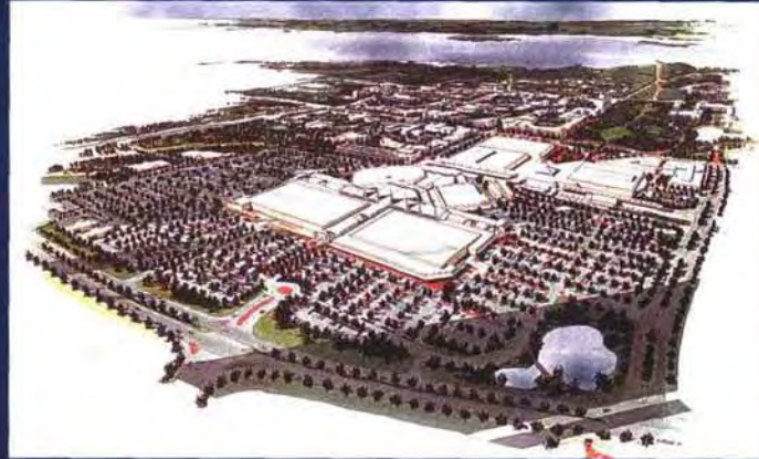
Shopping Centre Aerial
