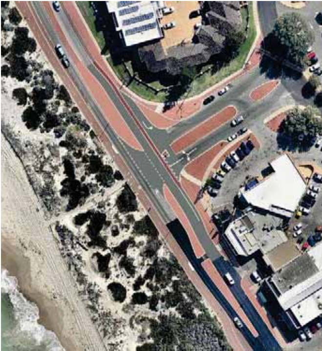
Figure 7-6 Mitigated West Coast Drive / The Plaza intersection with 6m wide central median
