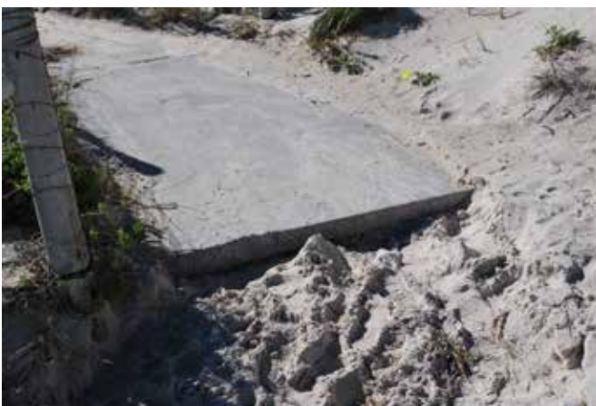
Figure 6: Erosion at the end of a concrete path and on higher foredunes in the south-west of the Reserve
