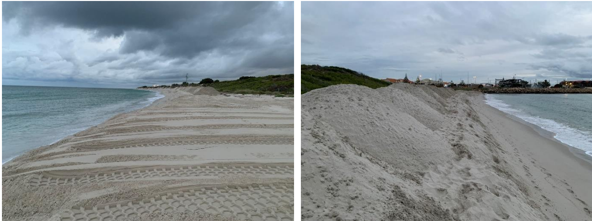
Figure 6.4 L) Disposal Area Looking North; R) Disposal Area Looking South (2/4/20)
