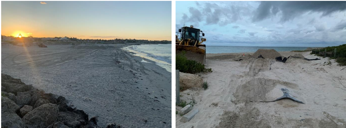
Figure 6.3 L) Extraction Area Looking South (26/3/20); R) Disposal Area Access Way (2/4/20)
