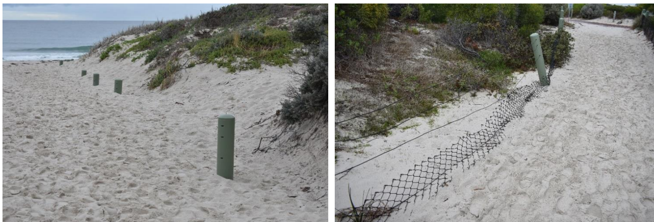
Figure 21: Fencing buried due to sand accretion on the beach and foredunes
