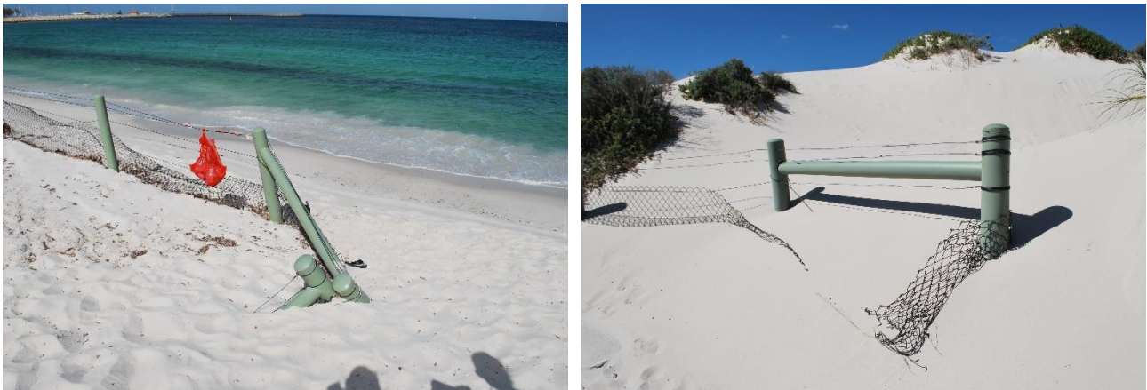
Figure 6: Erosion along the foredunes and beach affecting stability of fencing
