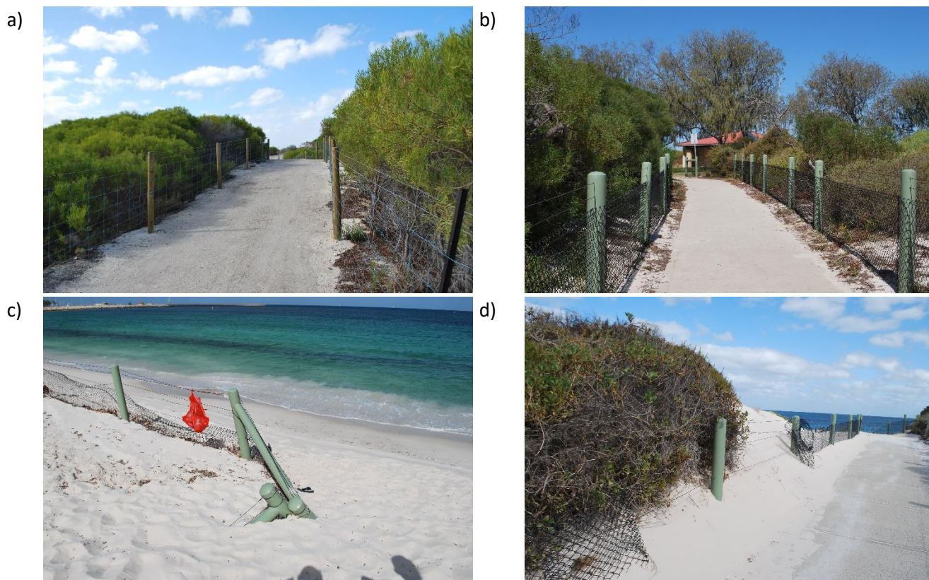
Figure 21: Fencing: a) pine post and square ringlock and wire fencing, b) PVC sleeves over pine posts and chainmesh fencing, c) fencing buried due to coastal erosion of sand dunes, d) fencing damaged along beach access path.
