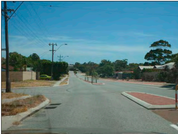
Photo 1: Camberwarra Dr, looking west towards Fenellia Cres
