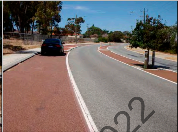
Photo 10: Approximate sight lines from Road 1 along Camberwarra Dr to the east
