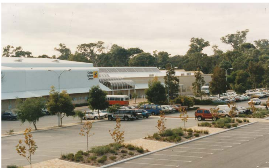
P00424.01 Craigie Leisure Centre as viewed from the car park off Whitfords Avenue 1993.
