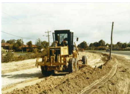
P02893 Construction of Whitfords Avenue ca. 1970.
