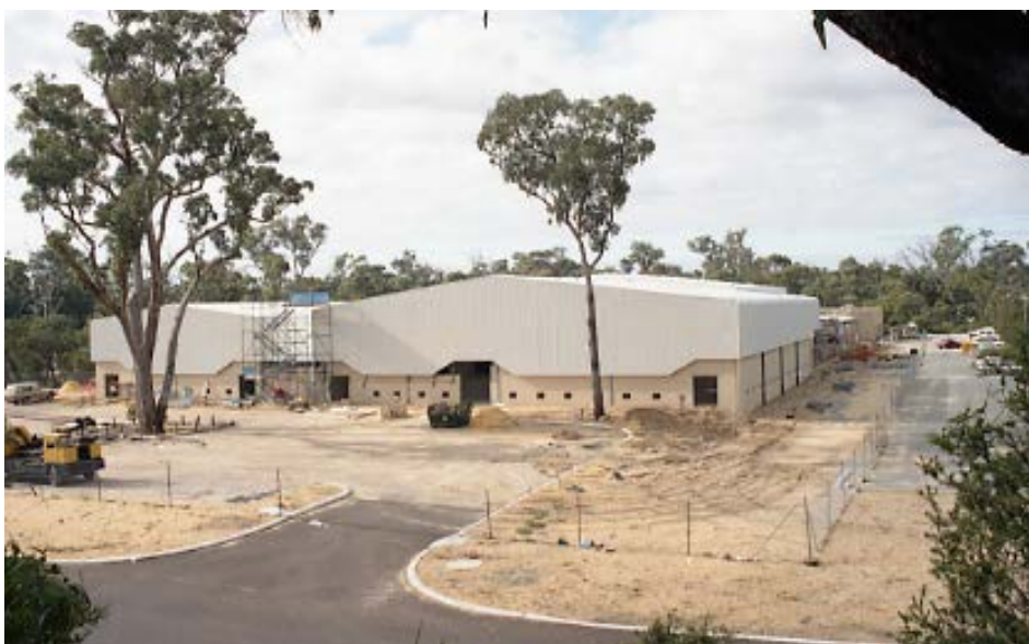
P01337.02 Craigie Leisure Centre under construction 1992.
