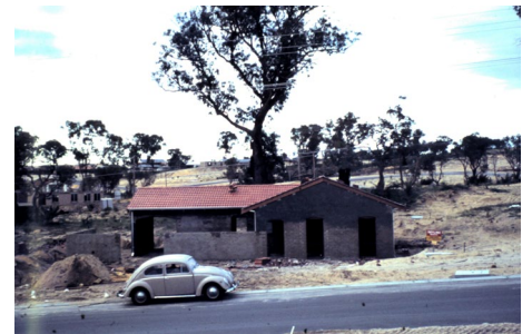
P03271.06: Home under construction at David Crescent Hillarys. 1972.
