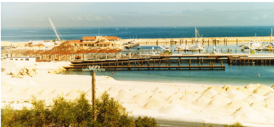
P02146.09: Hillarys Boat Harbour under construction, 1986.
