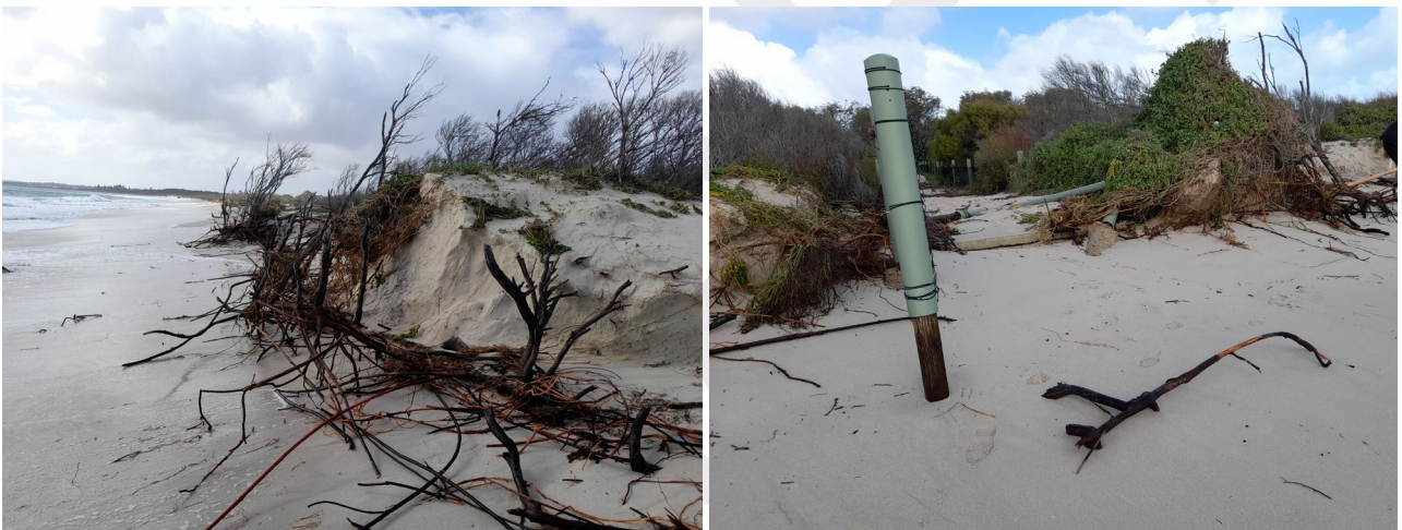
Figure 5-4 Eroded beach accessway and damaged dunes and vegetation at Pinnaroo Point, Hillarys (August 2022)
