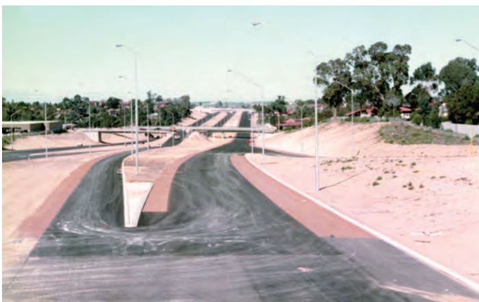
P01348.11 Road works - Mitchell Freeway. July 1986.
