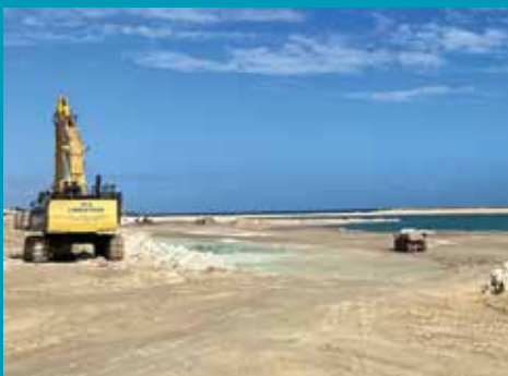
Caption: Construction continues at a fast pace.
