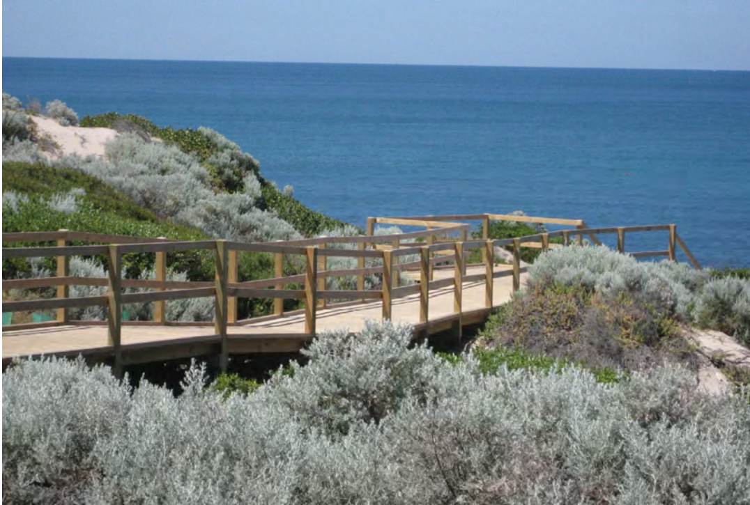
Figure 6: Stage 1 Boardwalk – Light impact construction over undulations and vegetation
