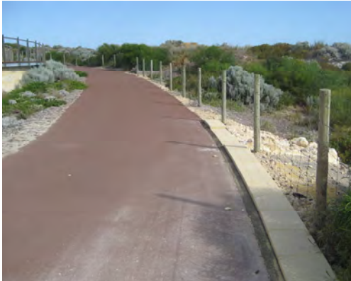
Figure 9: Stage 1 Dual Use Path – 3m wide red asphalt. Note limestone kerb to control minor drainage and galvanized wire and treated pine fencing to all sides(unless otherwise contained).
