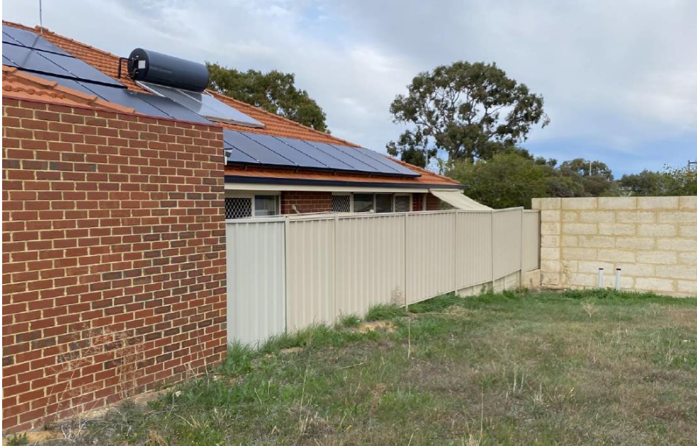
NORTHERN ELEVATION OF NO. 18
