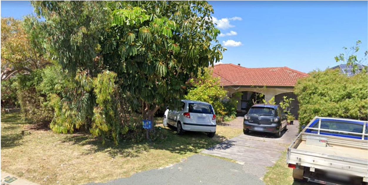
Figure 3 -Subject land and the existing dwelling that will be removed.
