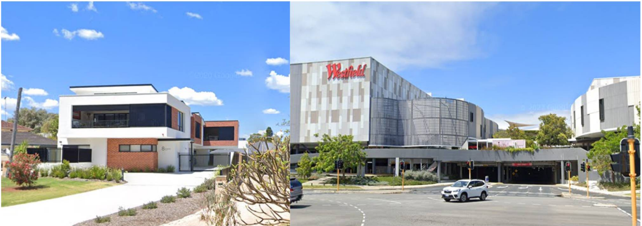
Figure 4 – The left photograph is of a new multiple dwelling development emerging within the area, whilst the right photograph represents the large bulkier shopping centre development.
