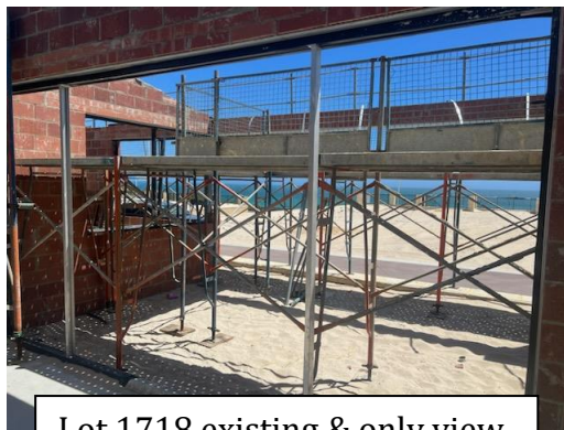
Lot 1718 existing & only view
