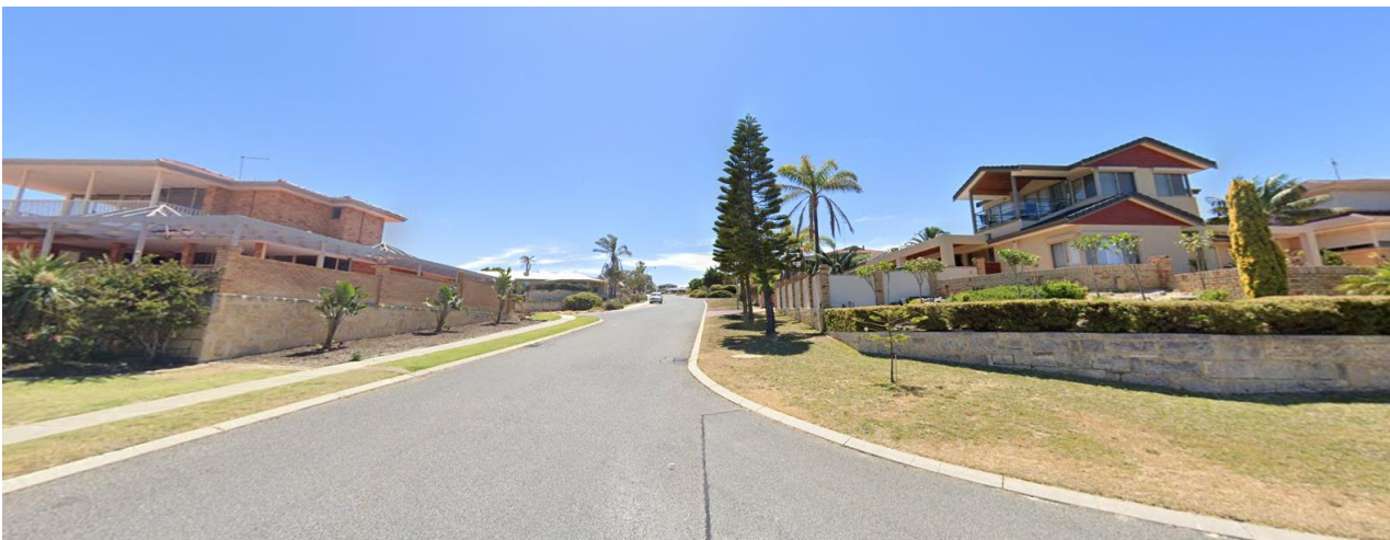
Figure 6 – Existing site works within the immediate streetscape.
