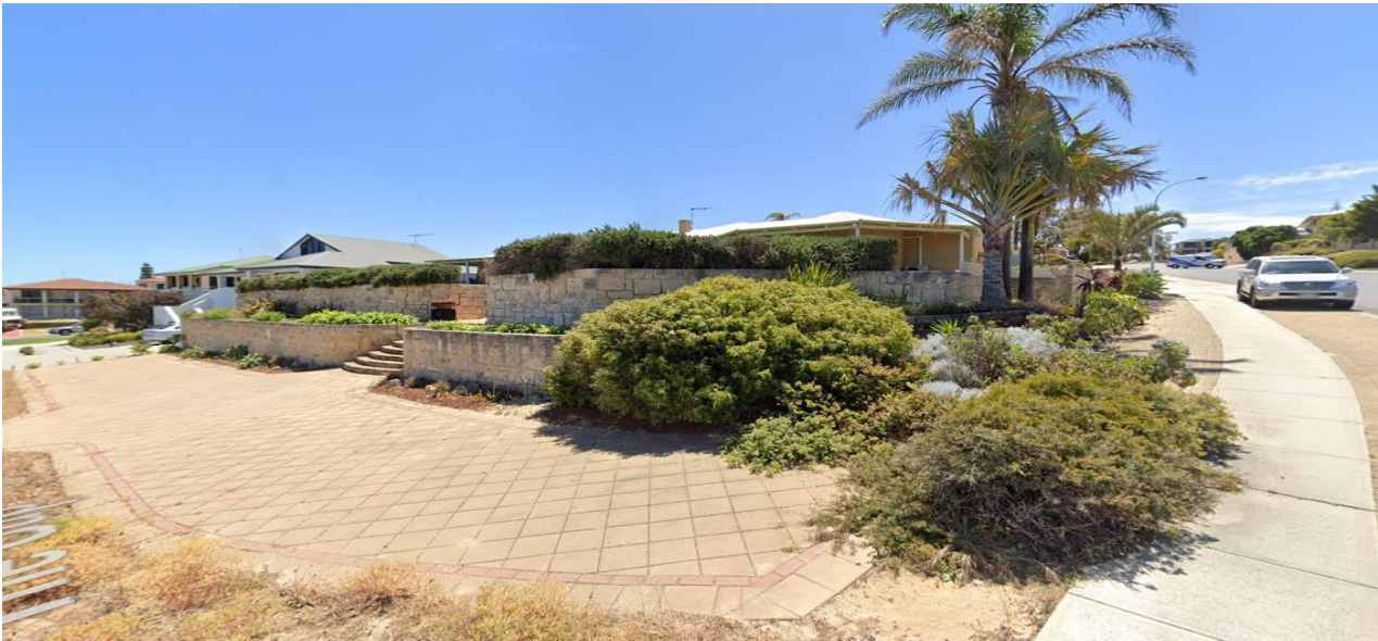
Figure 5 – Existing site works within the immediate streetscape.
