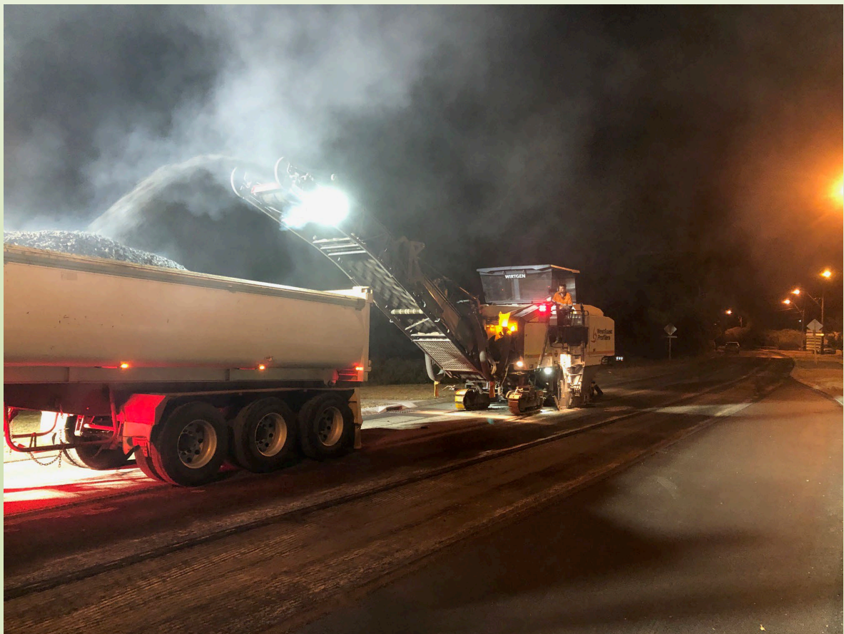
Road upgrade using recycled waste
